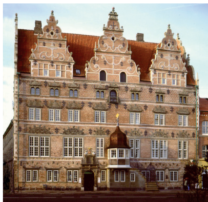
Photo of Jens Bang's House in the town of Aalborg from 1851. The house was built in the years 1623–1624 and has been the domicile for the Swan Pharmacy since 1665.
