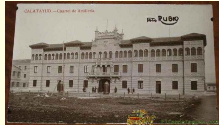
Military Pharmaceutical Complex of Calatayud (Zaragoza)
