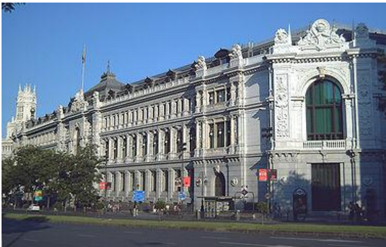
The Bank of Spain, the most influential body in the government's currency policy. North façade (Calle de Alcalá, street) of the Bank of Spain Building constructed between 1884 and 1891; extensions in 1930–35, 1969–75 and 2003–06.
